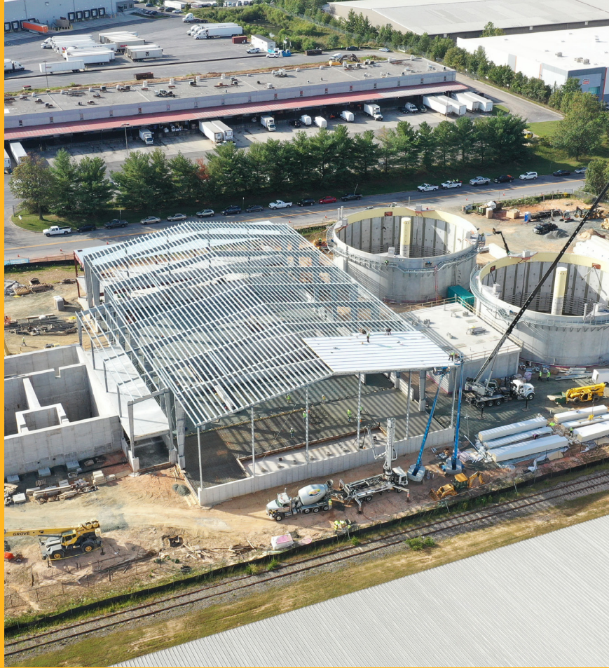
BioEnergy DevCo's food waste digester under construction at the Maryland Food Center Authority in Jessup.
