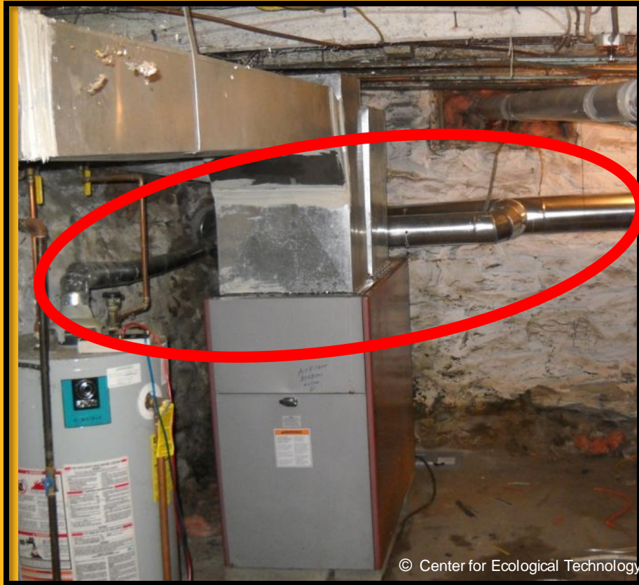
Long horizontal flue sections
