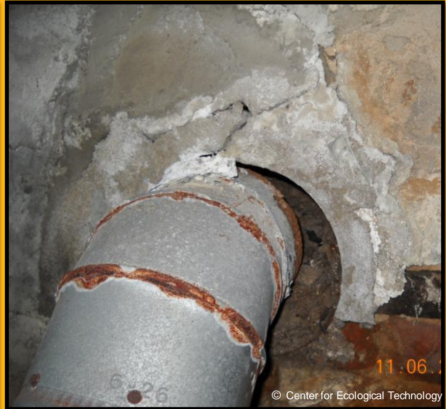
Poorly fitted flues
