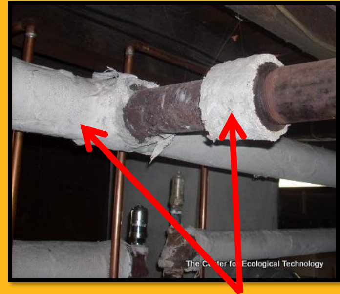
Asbestos on steam pipes
